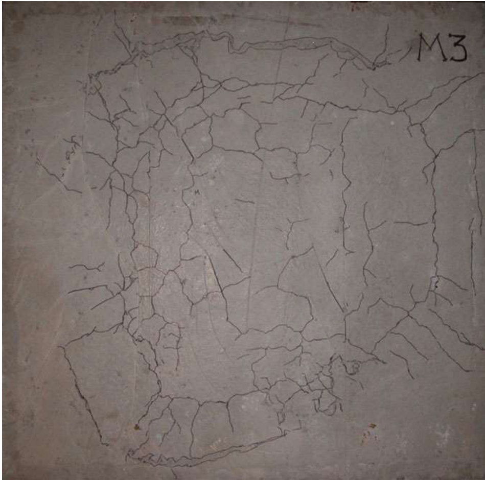
Fig. 3 Prototype in [7] after punching failure. Tensioned surface
